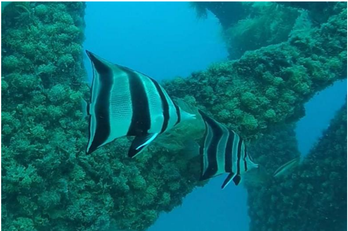
Figure 5. Assessment of the structural integrity.
